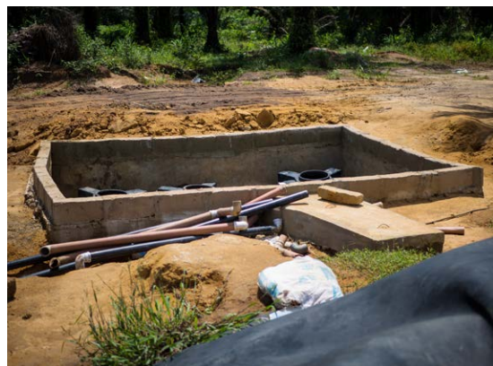
Lot 16: The sump is not covered so when it rains heavily it will fill up and overflow. Also pipes carrying water from the bio cell to the sump have failed. Water from the bio cell and sump flooded the surrounding environment after a recent rain incident. © Isaac Harry/cmapping.net Date: April 2020
