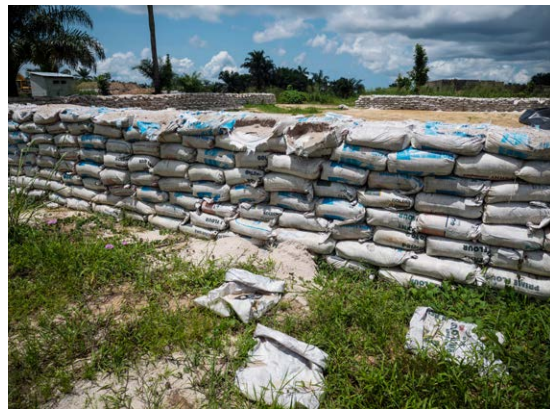
Lot 11: The bio cell has been partially constructed but the sand bags used for the bund wall are already torn, compromising its structural integrity. © Isaac Harry/cmapping.net Date: April 2020
