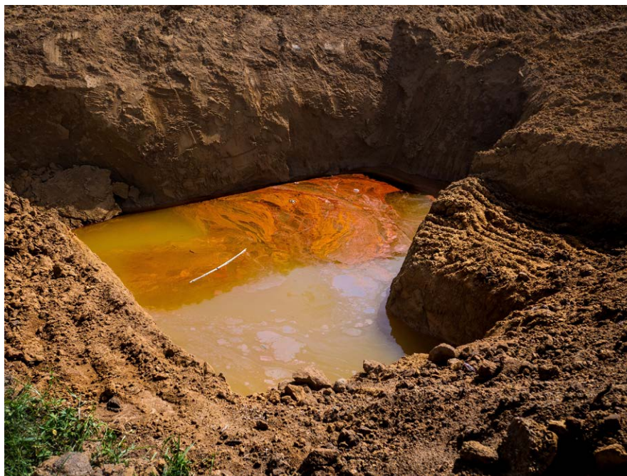
Lot 10: The excavated trench, with patches of oil and oxidized iron on groundwater. © Isaac Harry/cmapping.net Date: April 2020
